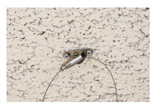
12. Attach the ceiling mounts to the ceiling. Then set the correct height of the fixture by pulling the wires through the ceiling mount. When the fixture height is correct, trim the excess mounting wire.
